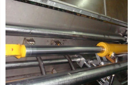
Packing drag test (with fully extended condition)
