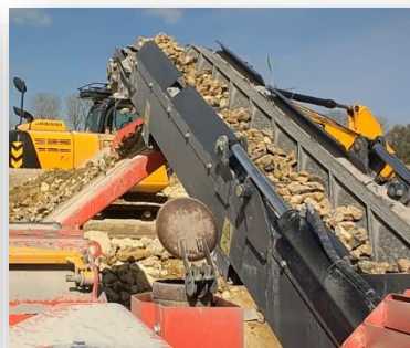
Oversize Material being returned to chamber
