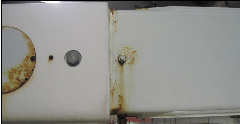
If corrosion progresses, the structural integrity of the boom is affected due to a reduction in the thickness of the material.
