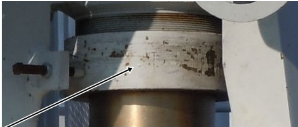
Packing Nut or Packing Gland
